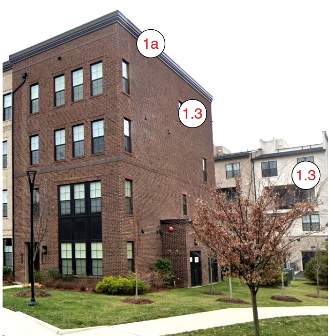
1.a FLAT ROOF with PARAPET Shed style roof is concealed by the parapet at front & side (shed at back is exposed)
