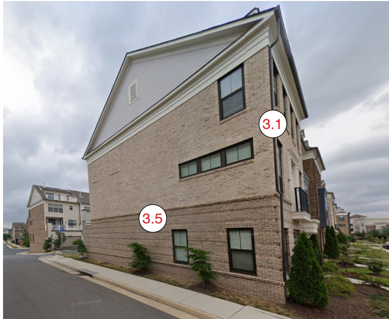
All materials turn the outside corner and extend at least 2ft or 2ft beyond openings; horizontal transition is extended at least 2ft above the openings
