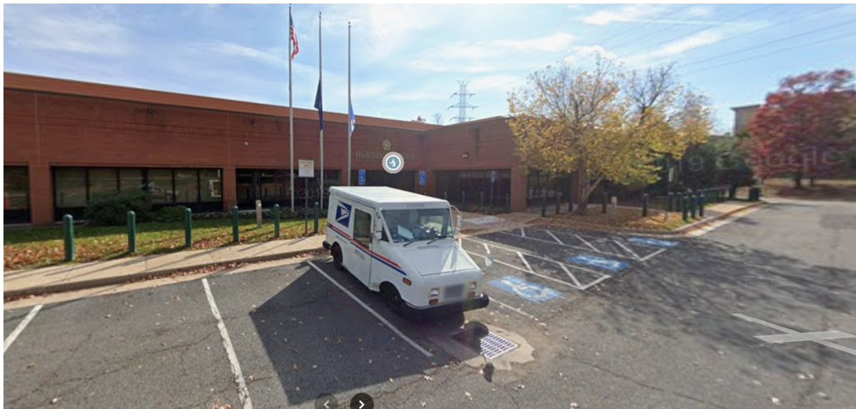
Figure 3: HPD Building, note that the brick is an orange-red color (image source: Google).
