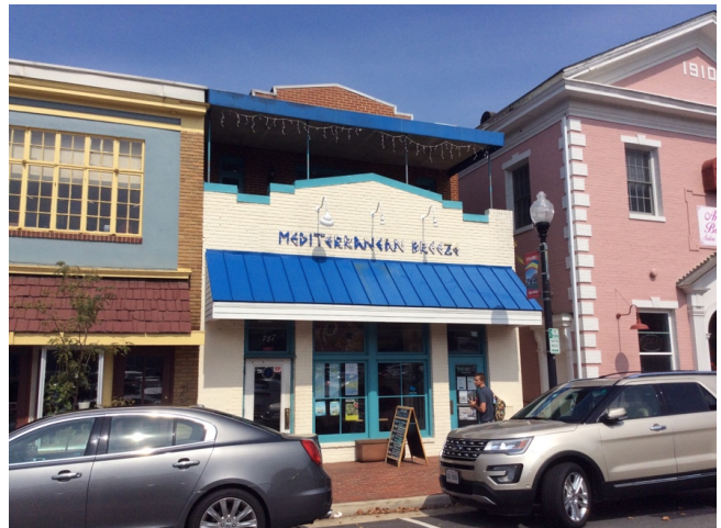
Photograph - Primary Elevation(s)
