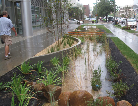
Bioretention bioswale on sidewalk, Baltimore, MD
