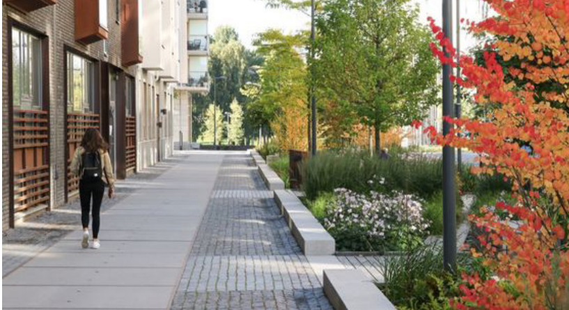
Pervious pavers demarcating entryways and pedestrian circulation next to fully grown rain garden
