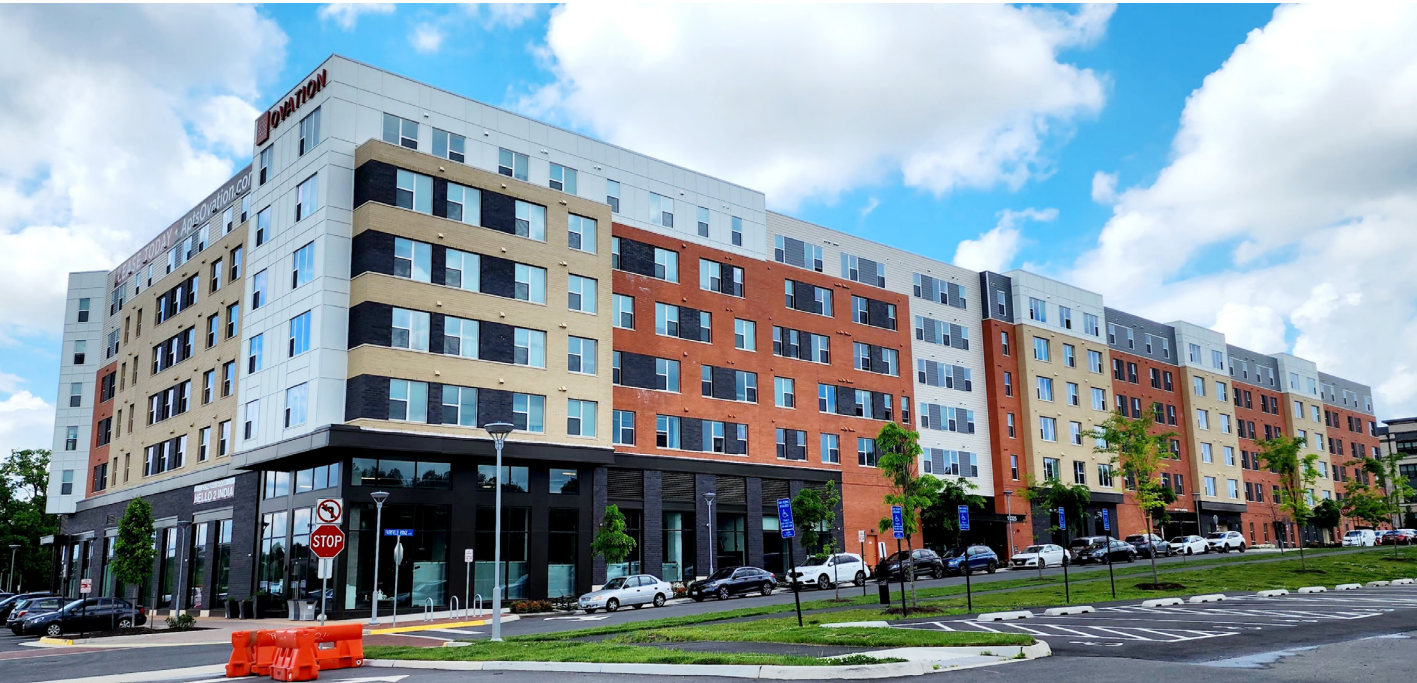
The Ovation at Arrowbrook, a Fairfax County affordable housing project with 274 apartment units serving households earning 30% to 60% of the average median income
