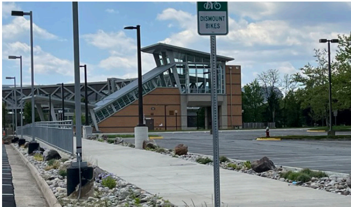
13 HERNDON METRO STATION
