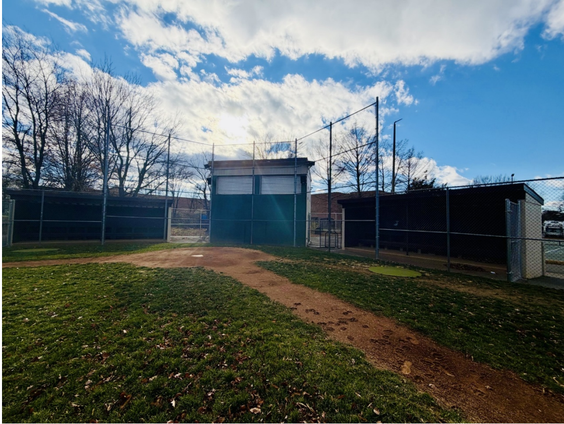
Figure 2: Dugouts at Bready Park with press box in center. December 2025
