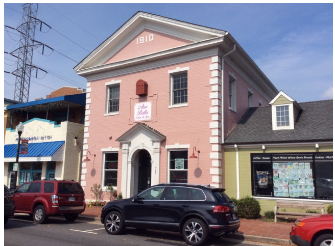
Photograph - Primary Elevation(s)
