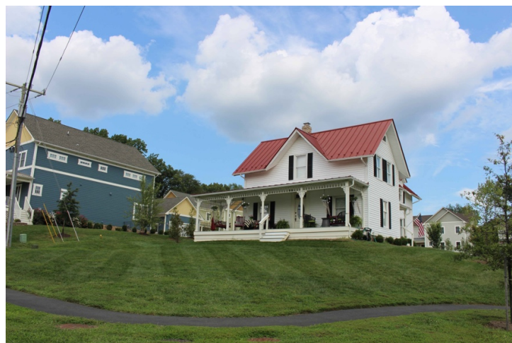
Photograph - Primary Elevation(s)
