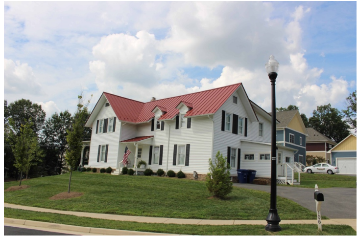
Photograph - Secondary Elevations or Details
