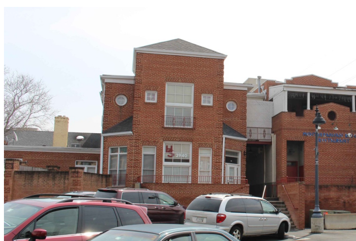
Photograph - Secondary Elevations or Details
