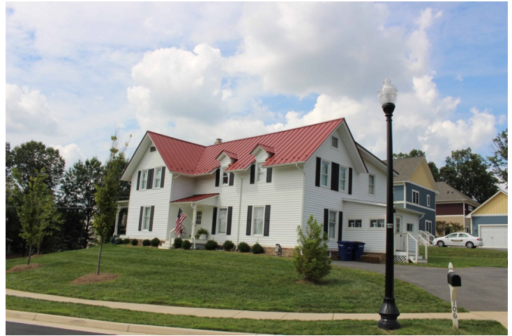
Photograph - Secondary Elevations or Details
