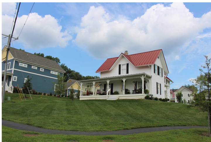
Photograph - Primary Elevation(s)
