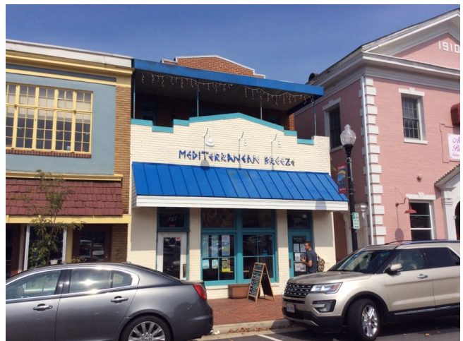
Photograph - Primary Elevation(s)
