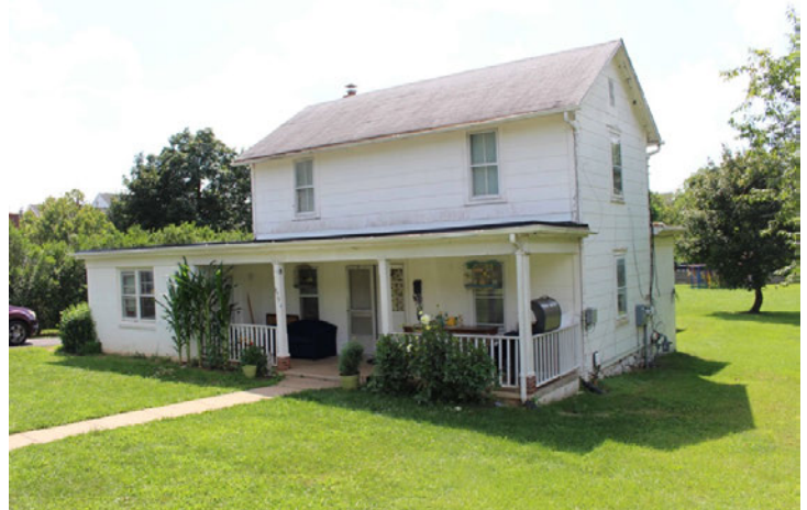
Photograph - Primary Elevation(s)
