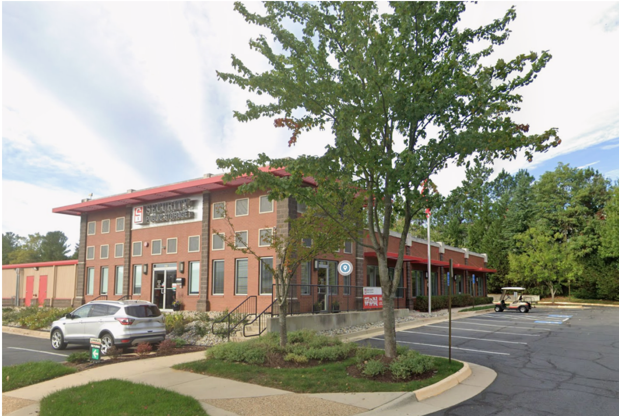
Figure 3: Storage facility at 385 Spring Street to the west of the subject property. Note the use of masonry on the façade.
