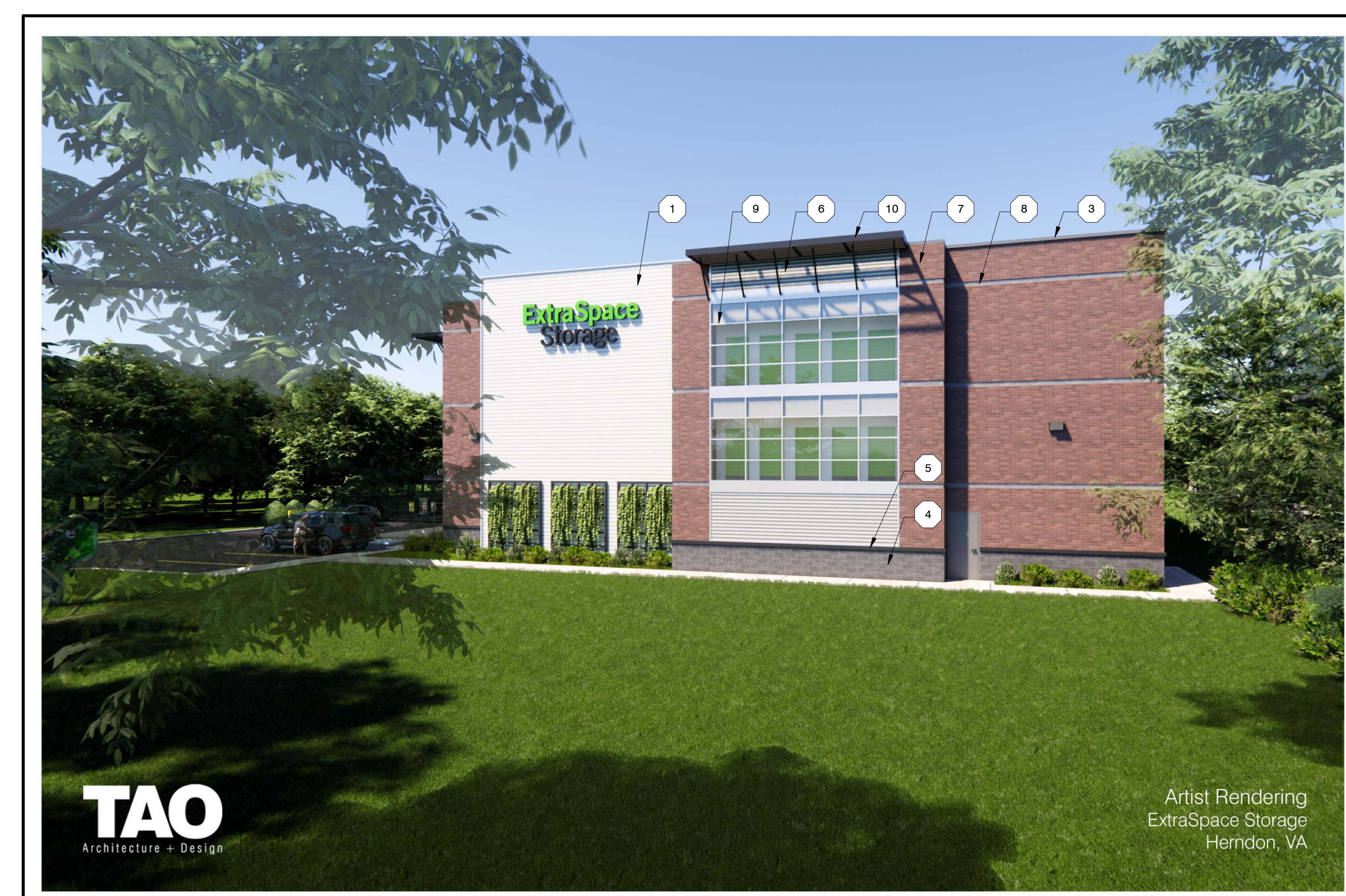
SOUTH EAST CORNER
