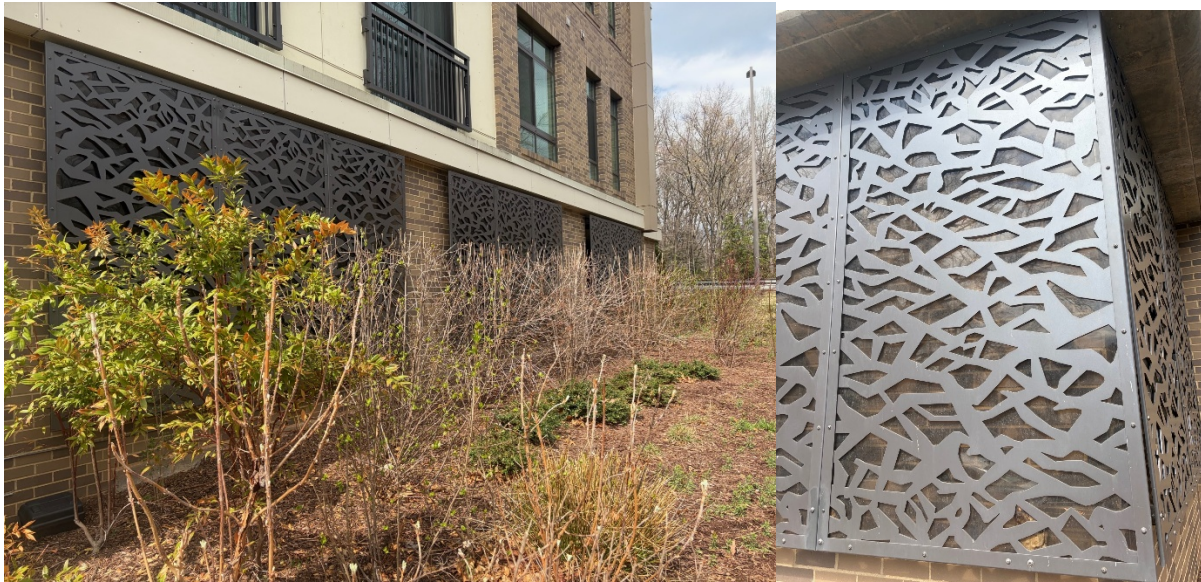
Figure 3: Example of a garage screen that obstructs view of the parking structure (located at 11444 N Shore Dr, Reston, VA 20190).
