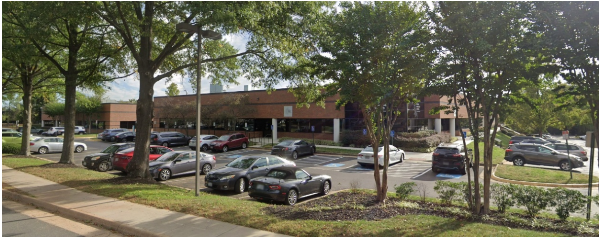
Figure 4: Office building at 450 Springpark Place to the west of the subject property that employs a mix of glazing, masonry, and storefront systems along the façade.
