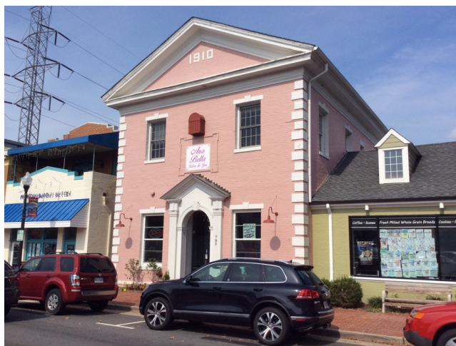
Photograph - Primary Elevation(s)
