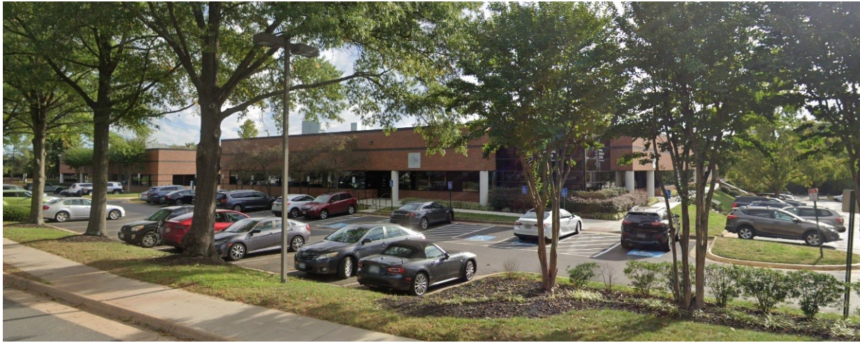
Figure 4: Office building at 450 Springpark Place to the west of the subject property that employs a mix of glazing, masonry, and storefront systems along the façade.
