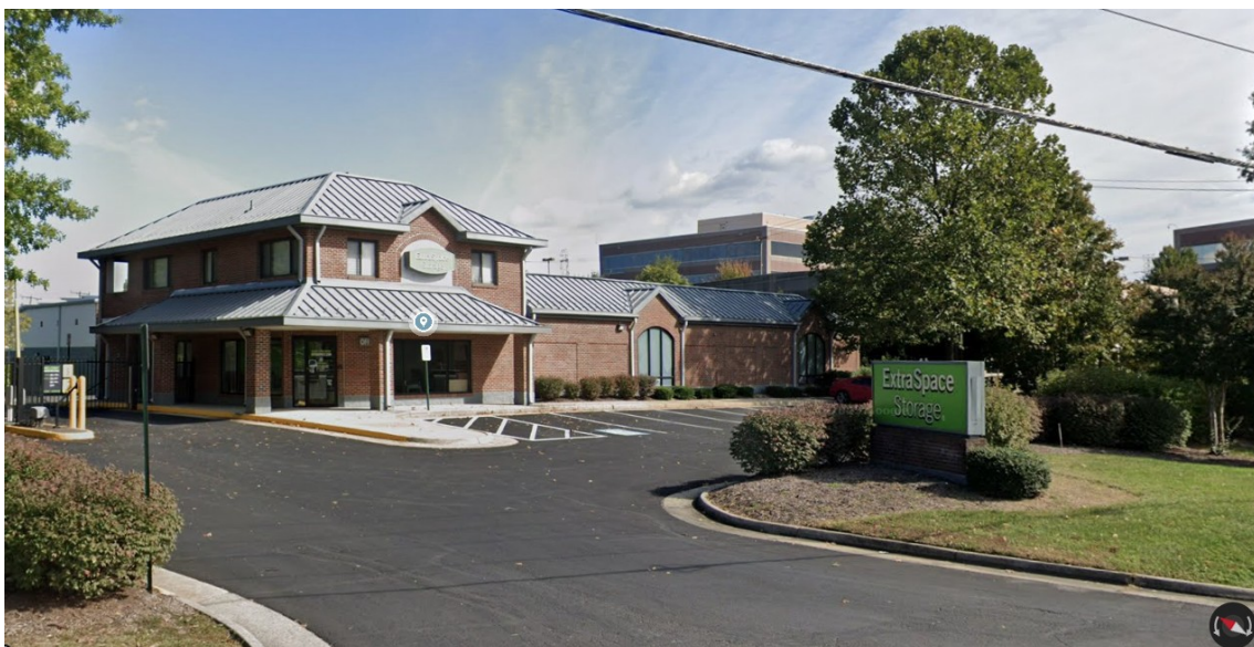
Figure 1: Present-day design of self-storage office viewed from the right-of-way.
