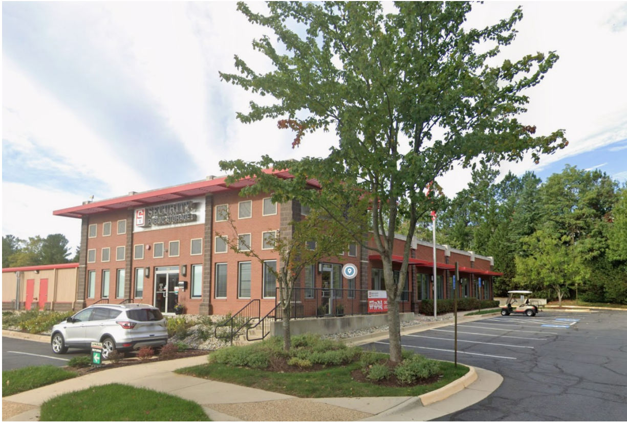
Figure 3: Storage facility at 385 Spring Street to the west of the subject property. Note the use of masonry on the façade.
