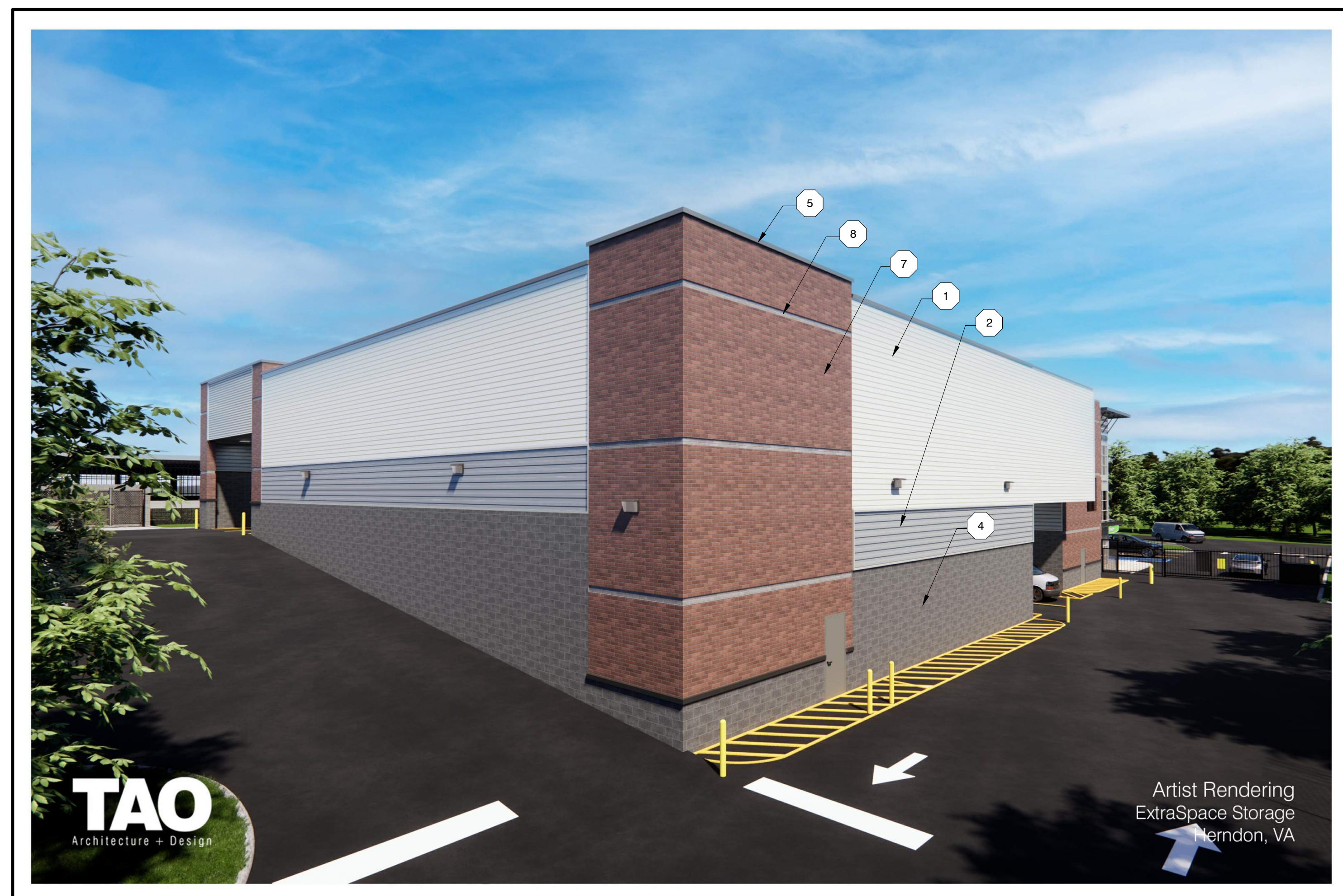
NORTHWEST CORNER VIEW
