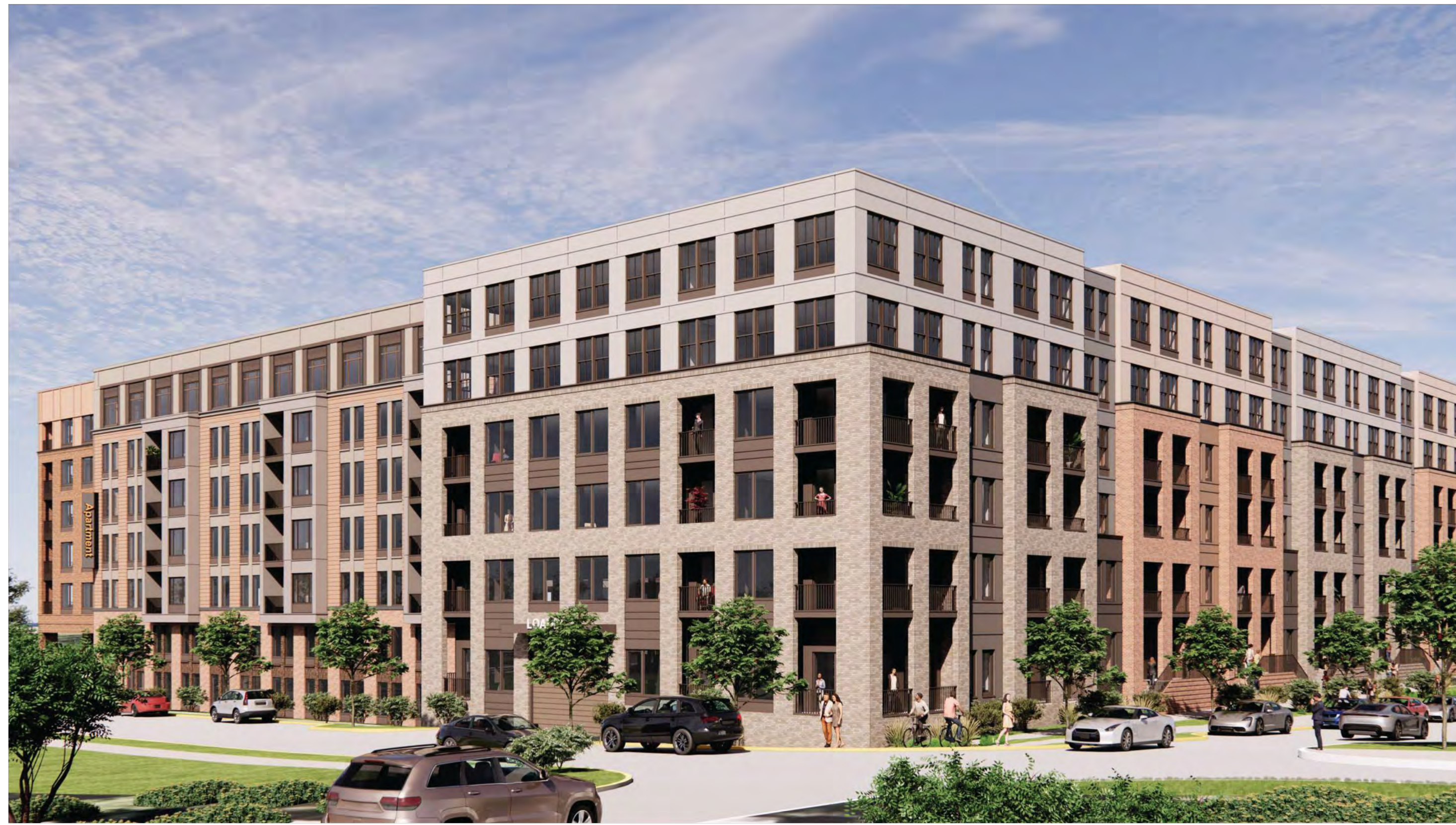
03 NE CORNER LOOKING WEST
