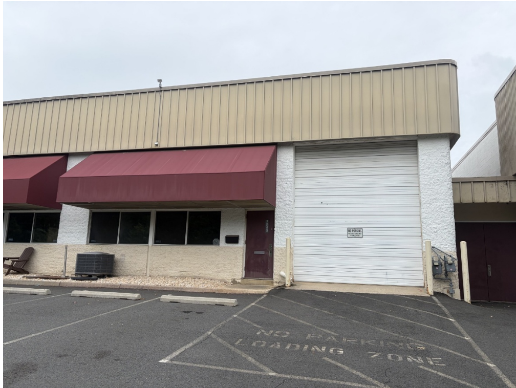
Figure 1: Photograph showing existing conditions at 259 Sunset Park Drive.
