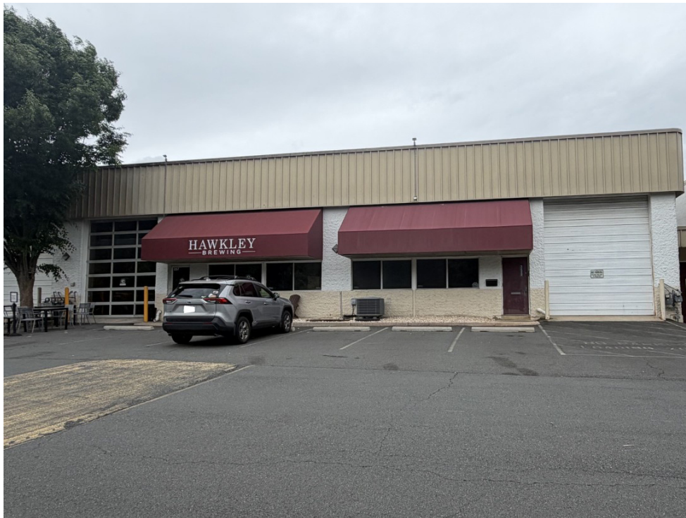
Figure 2: Photograph showing existing conditions at 259 Sunset Park Drive and adjacent property 257 Sunset Park Drive.
