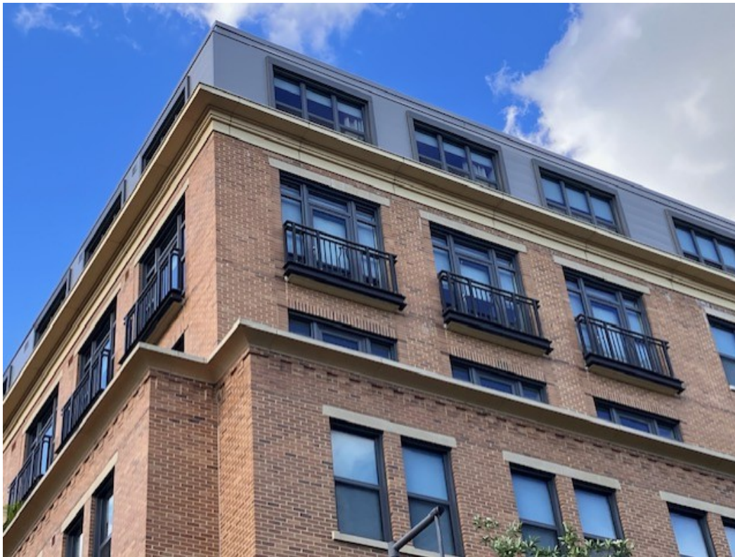
Figure 2: Example of a building (located at 1111 Belle Pre Way, Alexandria, VA 22314) with a deep cornice that visually delineates the top of the building. It also demonstrates the use of a variety of material colors, details, and plane changes to break up the building mass along the street.
