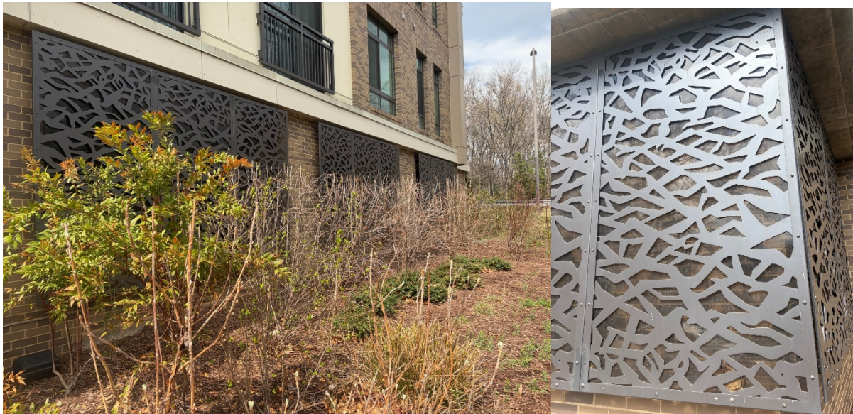
Figure 3: Example of a garage screen that obstructs view of the parking structure (located at 11444 N Shore Dr, Reston, VA 20190).
